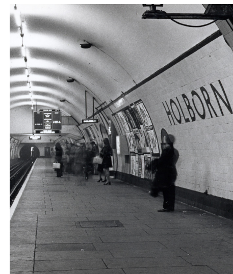
Central line platforms at Holborn
