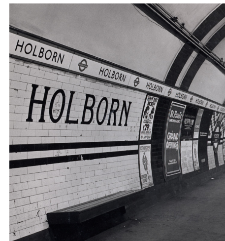
Piccadilly line platforms at Holborn, with original Leslie Green tiles
