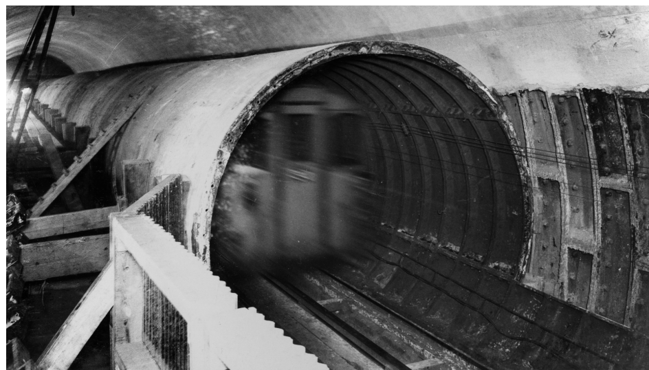
Central line platforms at Holborn
